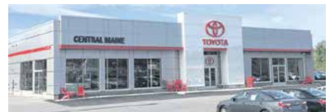
Central Maine Toyota 15 Airport Road, Waterville
